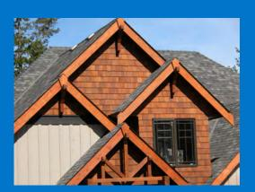
Watkins Sawmills Ltd. Appearance: Machine grooved for a shake texture from Number 1 Grade Blue Label CERTIGRADE
